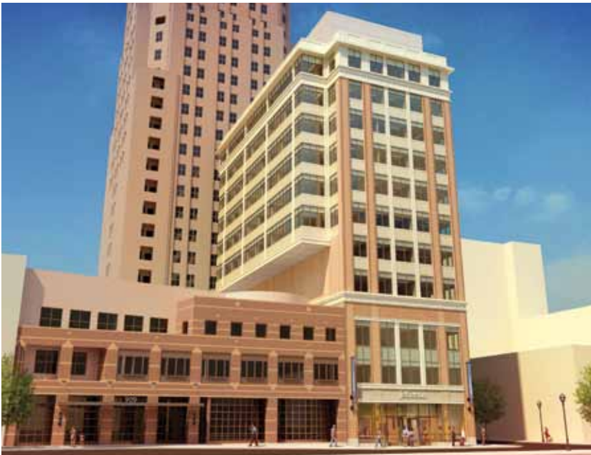
The new 21-story medical office building at Thomas Jefferson University, the largest freestanding academic medical center in Philadelphia, was designed to minimize disruption to occupants while allowing for phased expansion in the future. The project features architectural precast concrete panels on its façade, blending several colors and decorative styles to create visual interest and emphasize both horizontal and vertical features.
