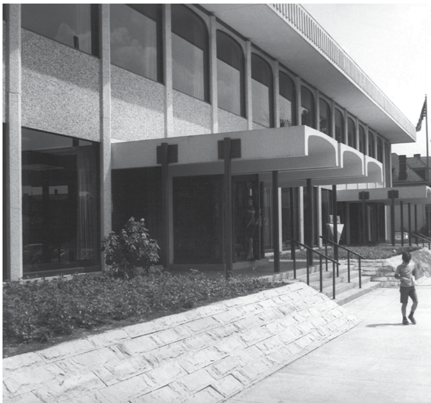
One of the first projects Kosar designed using precast concrete components was the YMCA in Butler, Pa. Completed in 1967, it features double tees spanning the natatorium as well as precast concrete components for the awnings over the entryway. Photos courtesy of Burt Hill, Inc.
